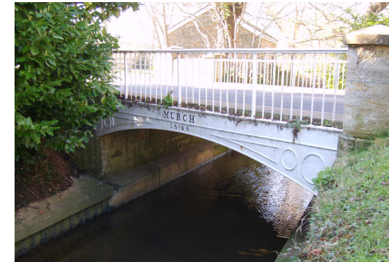
The grade 2 listed Hurst Bow Bridge from the Martock side. Made in 1843 in cast iron by Edward Murch, an ironfounder in Bridgwater. The other side of the bridge is Hurst.
