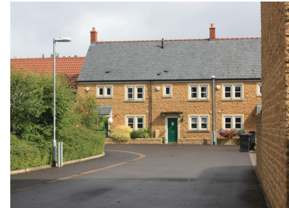
A modern terrace (2008). Well built with hamstone cladding and slate and tile mixed roof; it takes the eye round the corner. But the protruding window surrounds are crude heavy synthetic stone. The wooden double glazing frames cannot be as slender as the nineteenth century ones they are trying to match, but could still be far more elegant than these. Omitting the mullions, recessing the frames and painting them darker are simple ways of addressing these issues.
