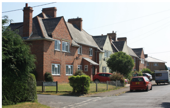
Two groups of four houses on Coat Road, brick built probably before the First War by architects Petter and Warren with a clear Arts and Crafts influence. The forward facing gables add interest as does the complex roof line with its characteristic dominant chimneys. The roof has an attractive variation in pitch just above the gutter and extends down to the first floor at the back.
